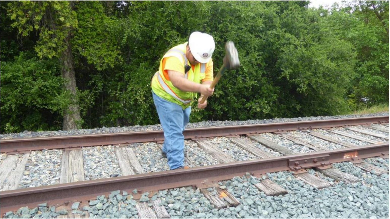
Anthony knocks out a couple rail-anchors
