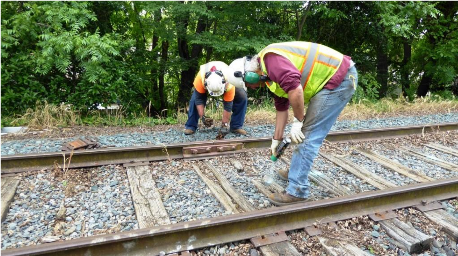
Steve continues marking bad ties while Mike F. collects spikes and tie-plates
