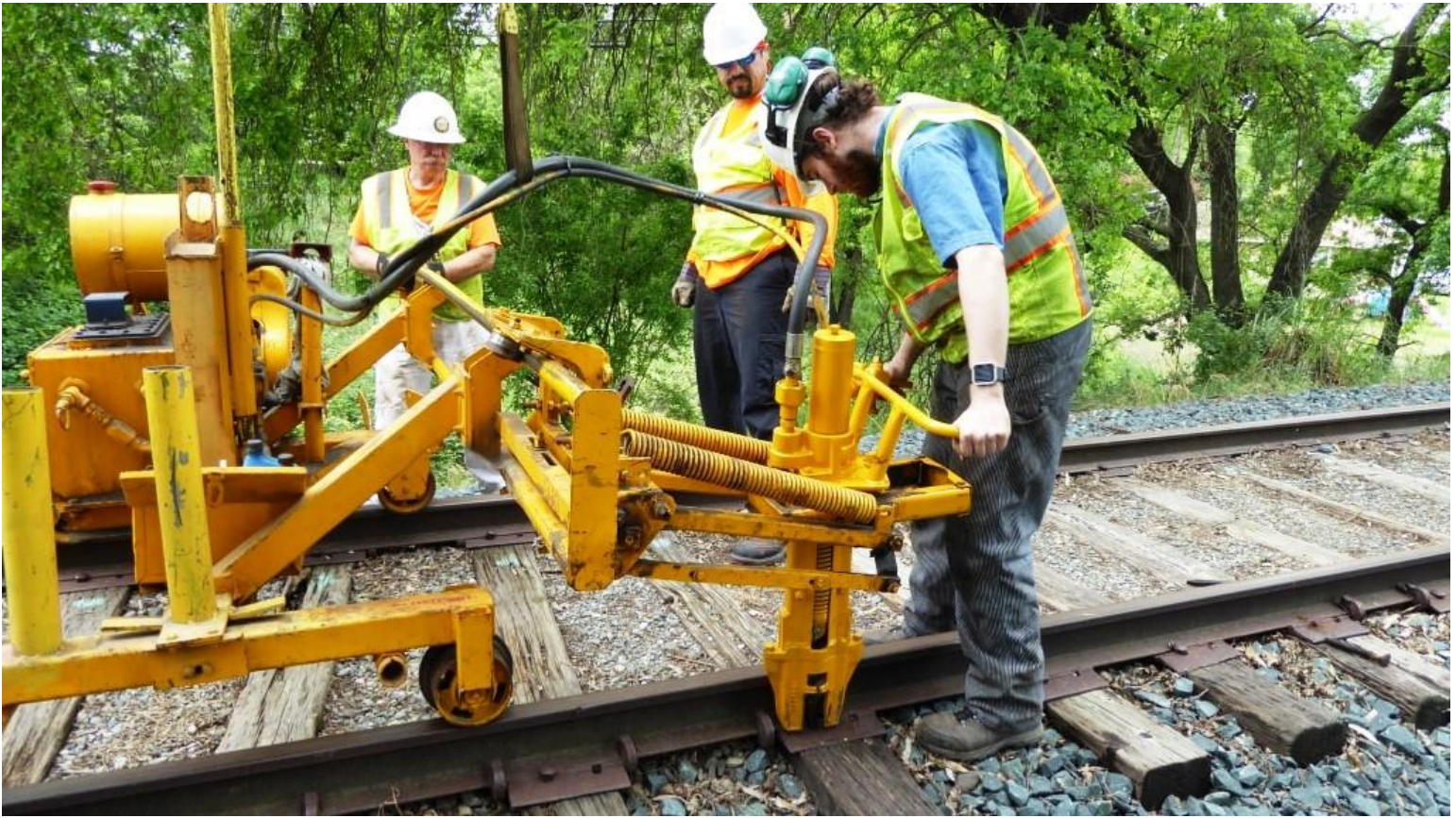
Jose passes the puller's work-head over to Matt who pulled spikes on the east rail
