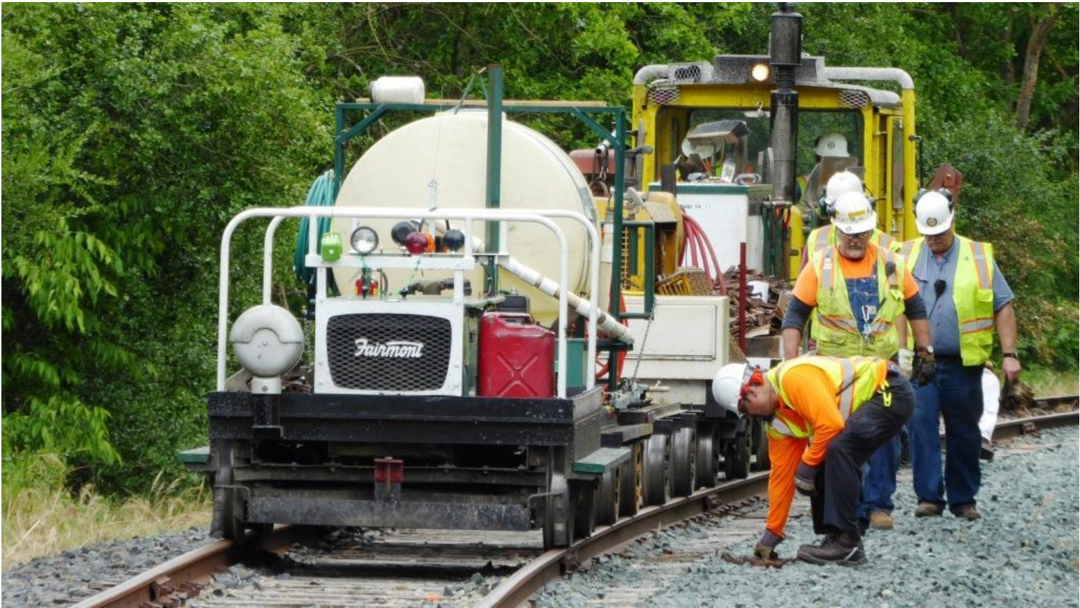
Heading back up the hill, Jose, Mike F., Steve, and Chris pick up spikes and tie-plates
