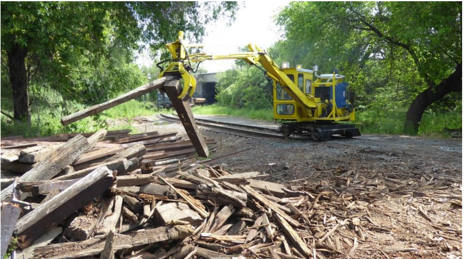
Alan in the tie-crane sorted solid tie pieces into piles for GM2 to pick up
