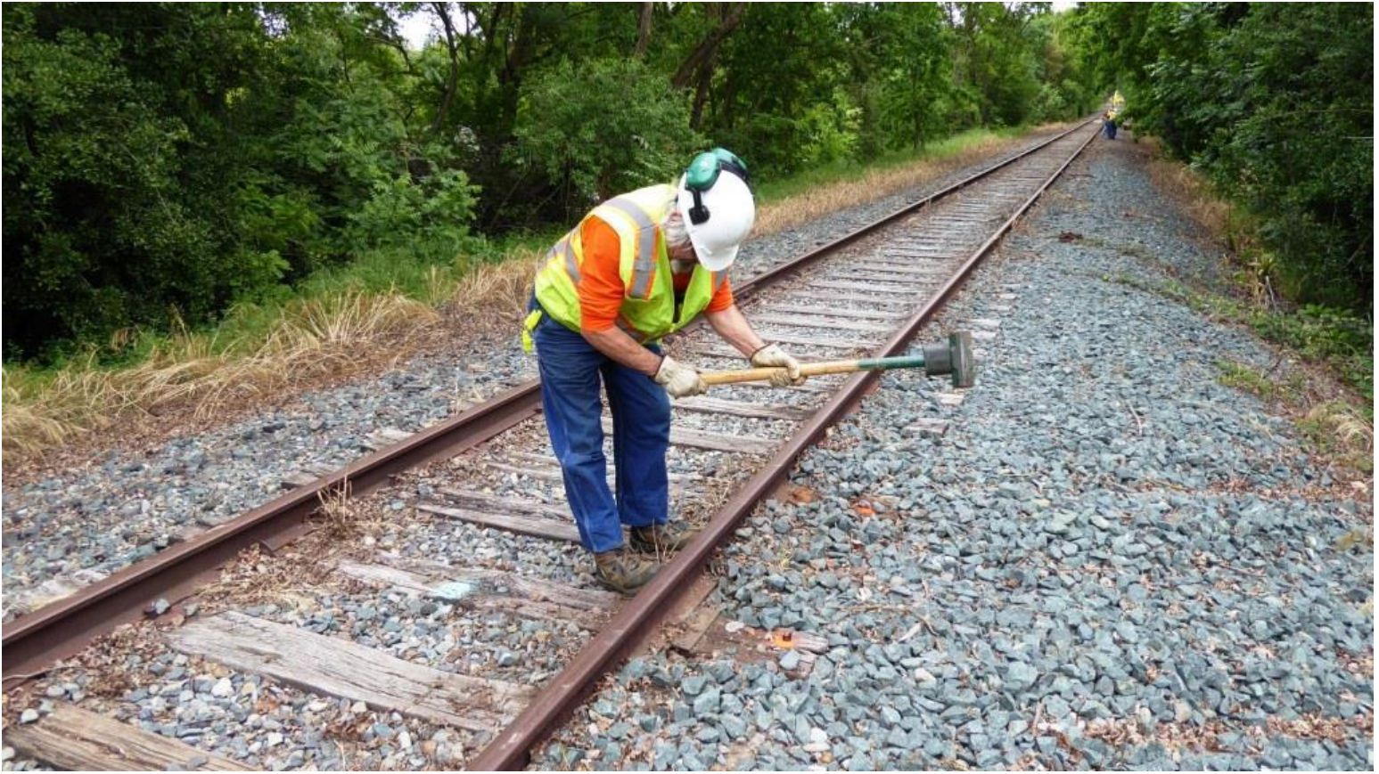
Ed knocks-out rail-anchors next to the ties being pulled
