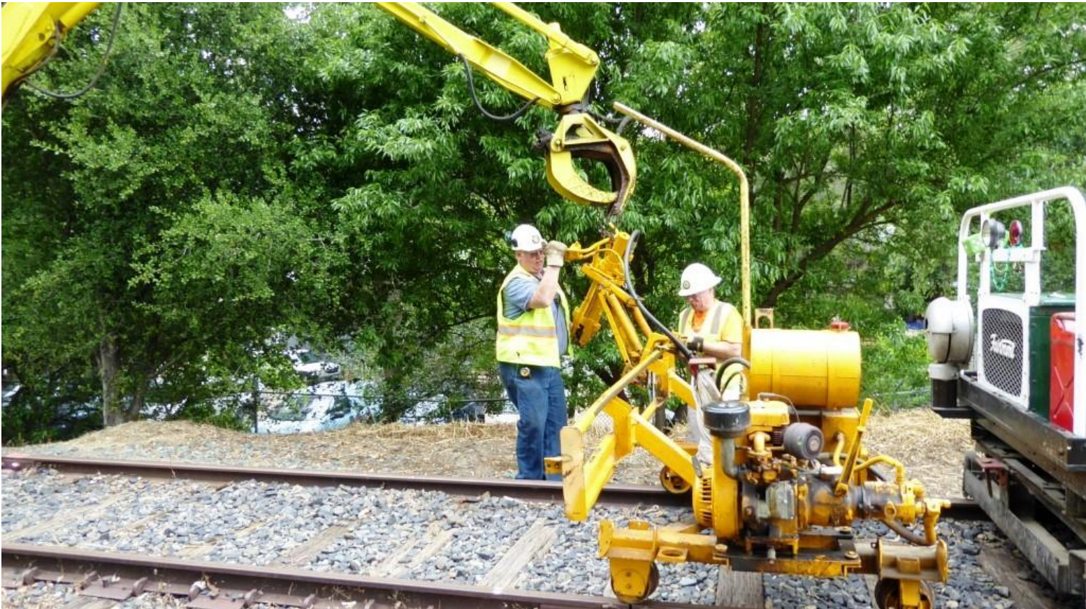
Time to put our toys away – Alan brings in the tie-crane to lift the spike-puller's work-head off to be stowed
