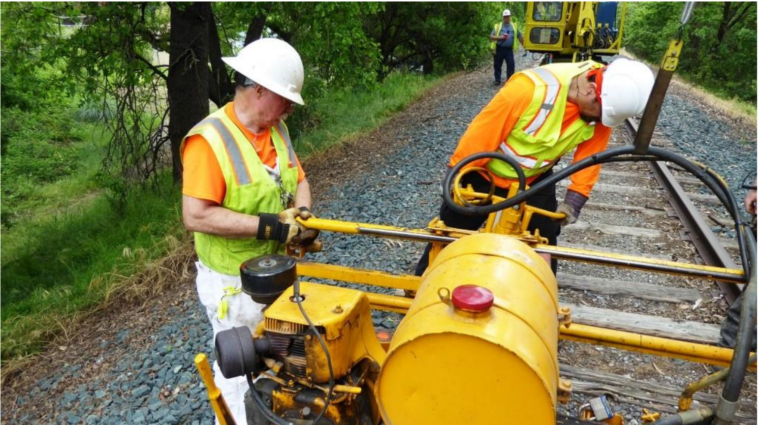
Now near the bottom of the hill, Mike H. and Jose keep right on pulling spikes
