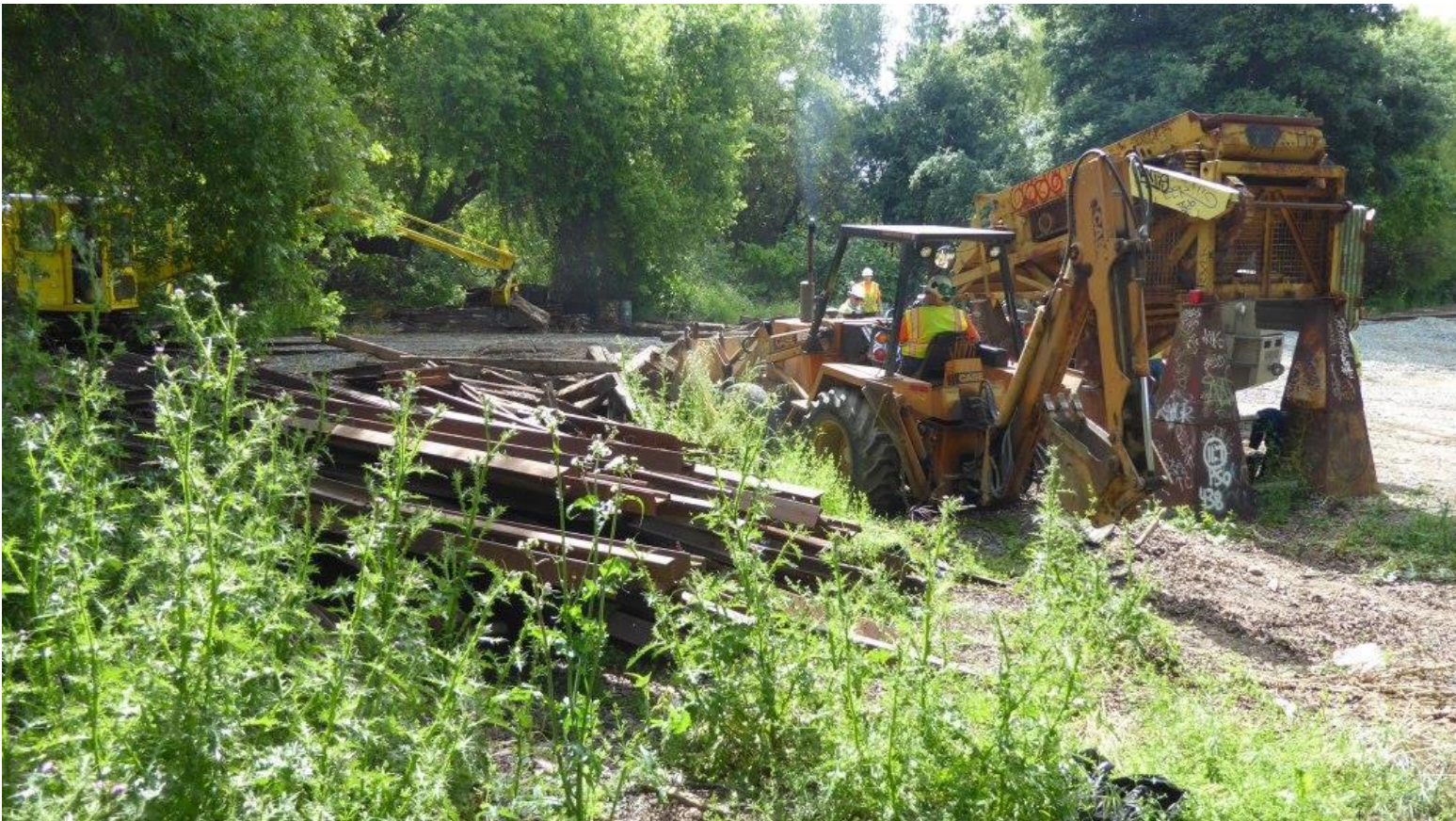
Harry brings the back-hoe in from the other side and scoops up a load of tie debris in the bucket
