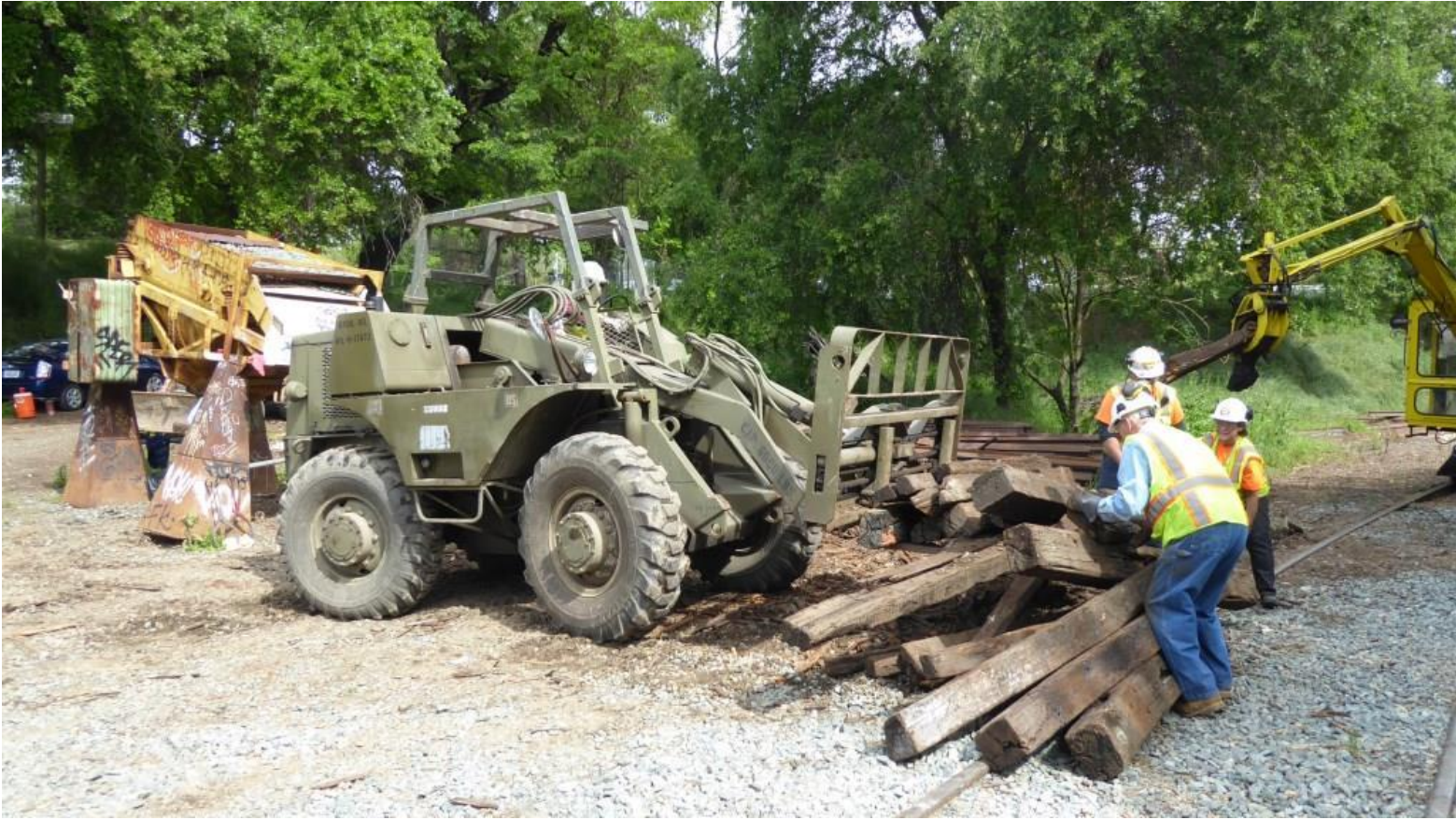
Steve grabs a pile of dead ties assisted by Clem, Pam, and Mike F.
