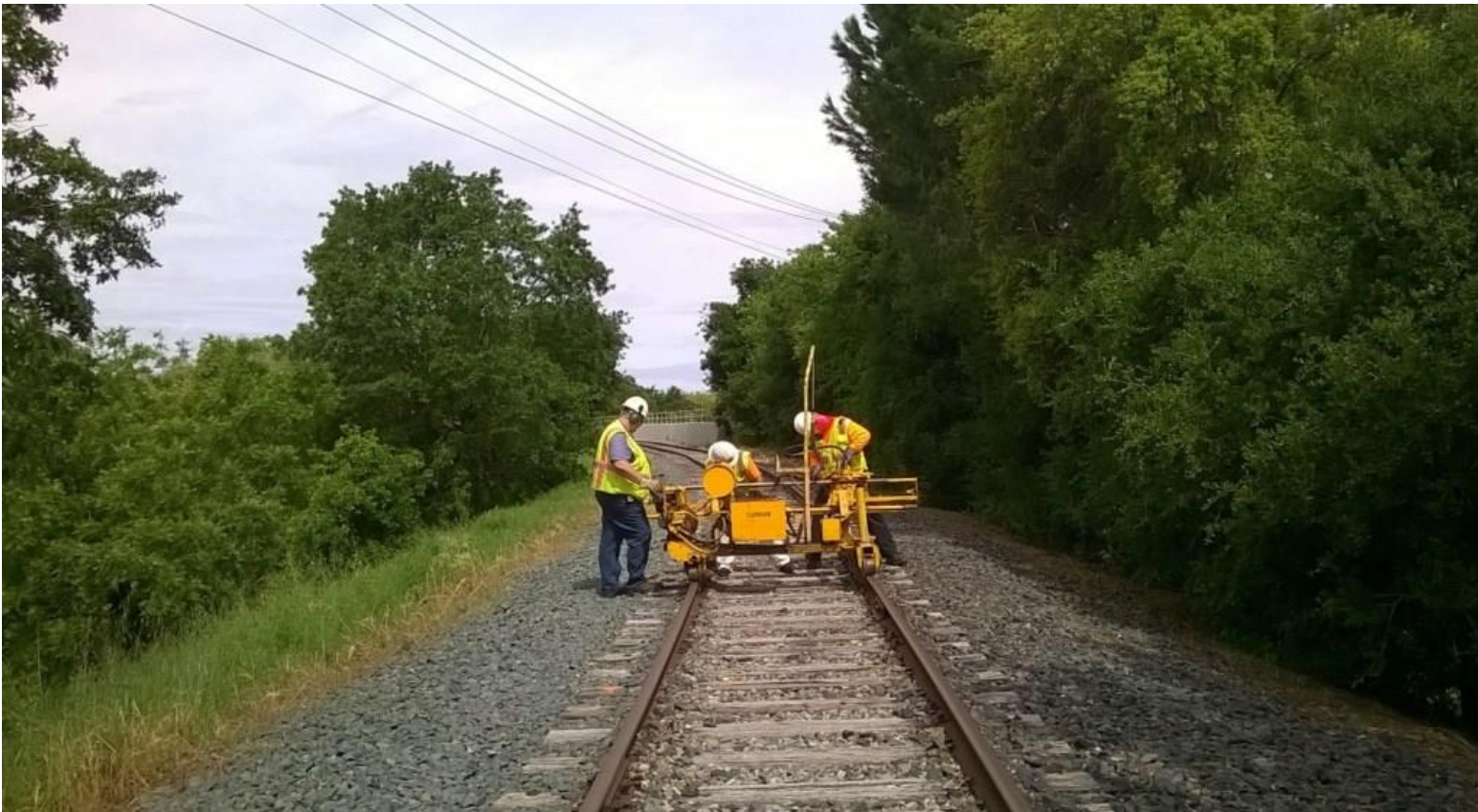
Slowly but surely, the spikes from 280 ties were pulled on Saturday
