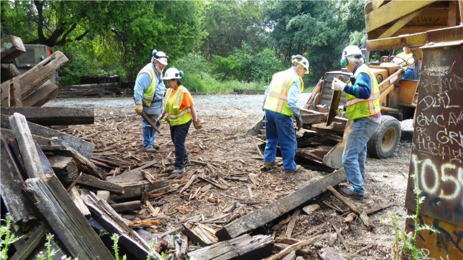
Frank, Pam, Clem, and Steve load the back-hoe's bucket with small tie debris
