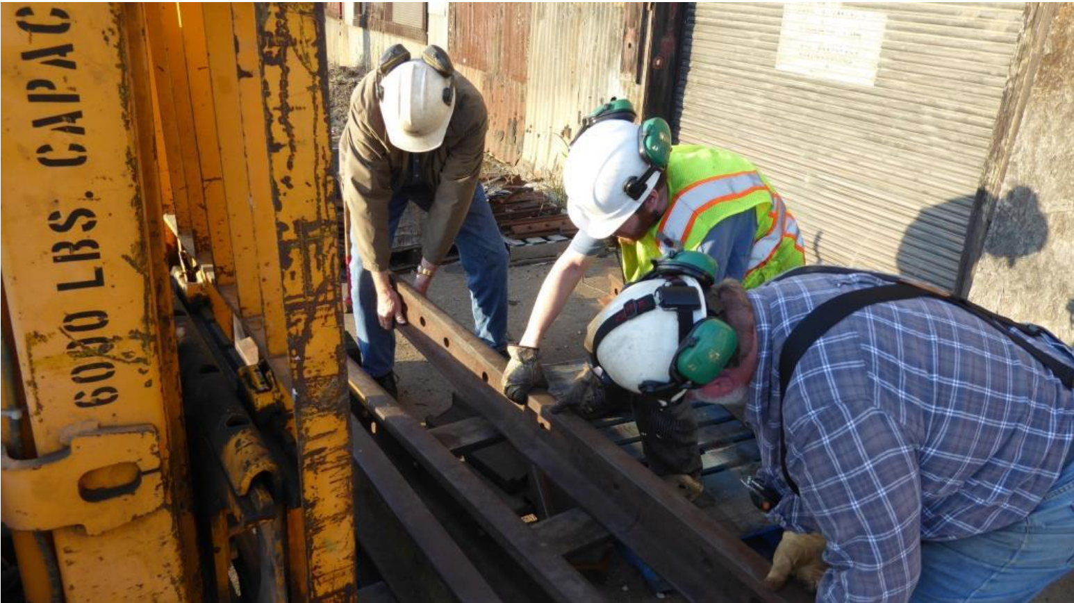
Alan, Matt, and Frank lift the wing-rail onto the forklift
