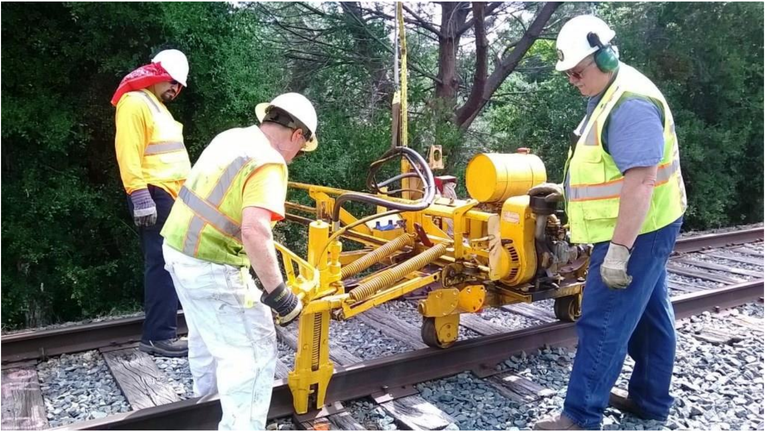
Working their way down the hill, Jose, Mike H., and Chris pull spikes
